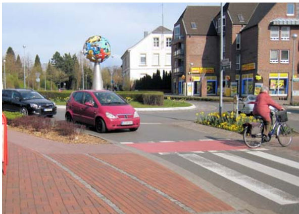
Figure 7 : Bicycle track combined with a zebra-crossing (urban, left) and combined with walkway (rural, right). In the urban context cyclists have the right of way whereas at rural intersections cyclists have to yield to motorized traffic.
