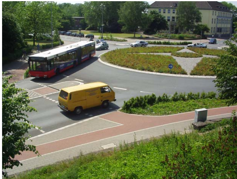
Figure 9 : Urban compact two-lane roundabout in Oberhausen
