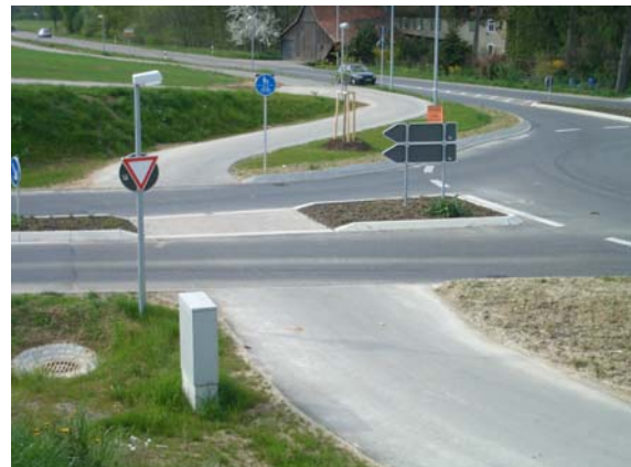
Figure 7 : Bicycle track combined with a zebra-crossing (urban, left) and combined with walkway (rural, right). In the urban context cyclists have the right of way whereas at rural intersections cyclists have to yield to motorized traffic.
