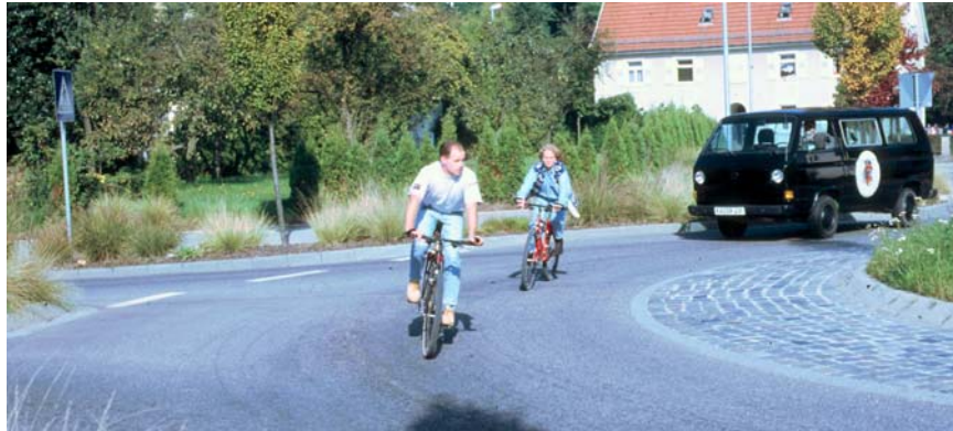
Figure 6 : Operation of bicycle traffic on the circular roadway for traffic volumes below an ADT of 15,000 veh/day. Due to similar desired speeds (in a range between 15 and 25 km/h) of cars and cyclists no overtaking is required. Cyclists can indicate their intended direction of driving clearly by their trajectory through the intersection.
