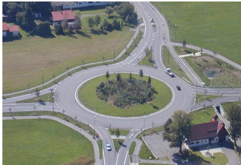
Figure 10 : Rural compact two-lane roundabout in Bad Aibling
