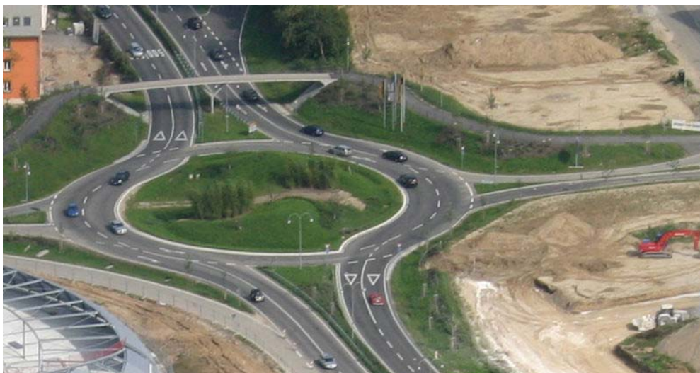
Figure 12 : Turbo-roundabout in Baden-Baden
